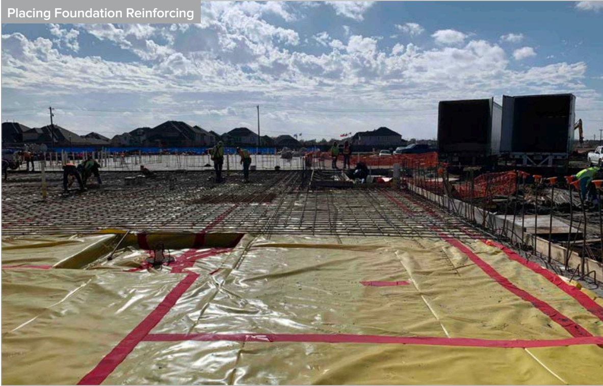
Placing Foundation Reinforcing
